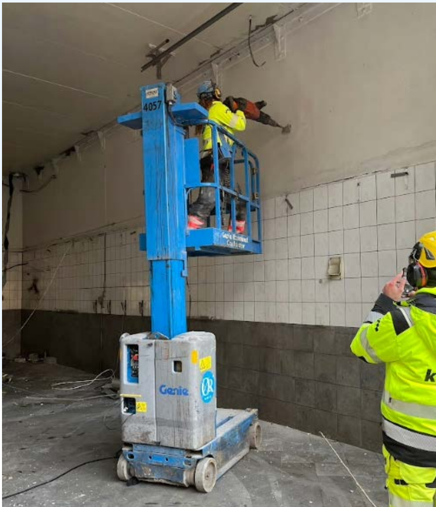
On-site testing of the in-situ concrete. Picture provided by Sirkulær Ressurssentral
